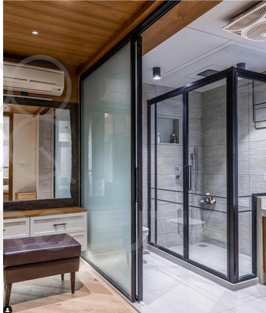
BATHROOM SLIDING PARTITION WITH FROSTED GLASS IN ZERO FRAME SUB-DIVIDING THE AREA
