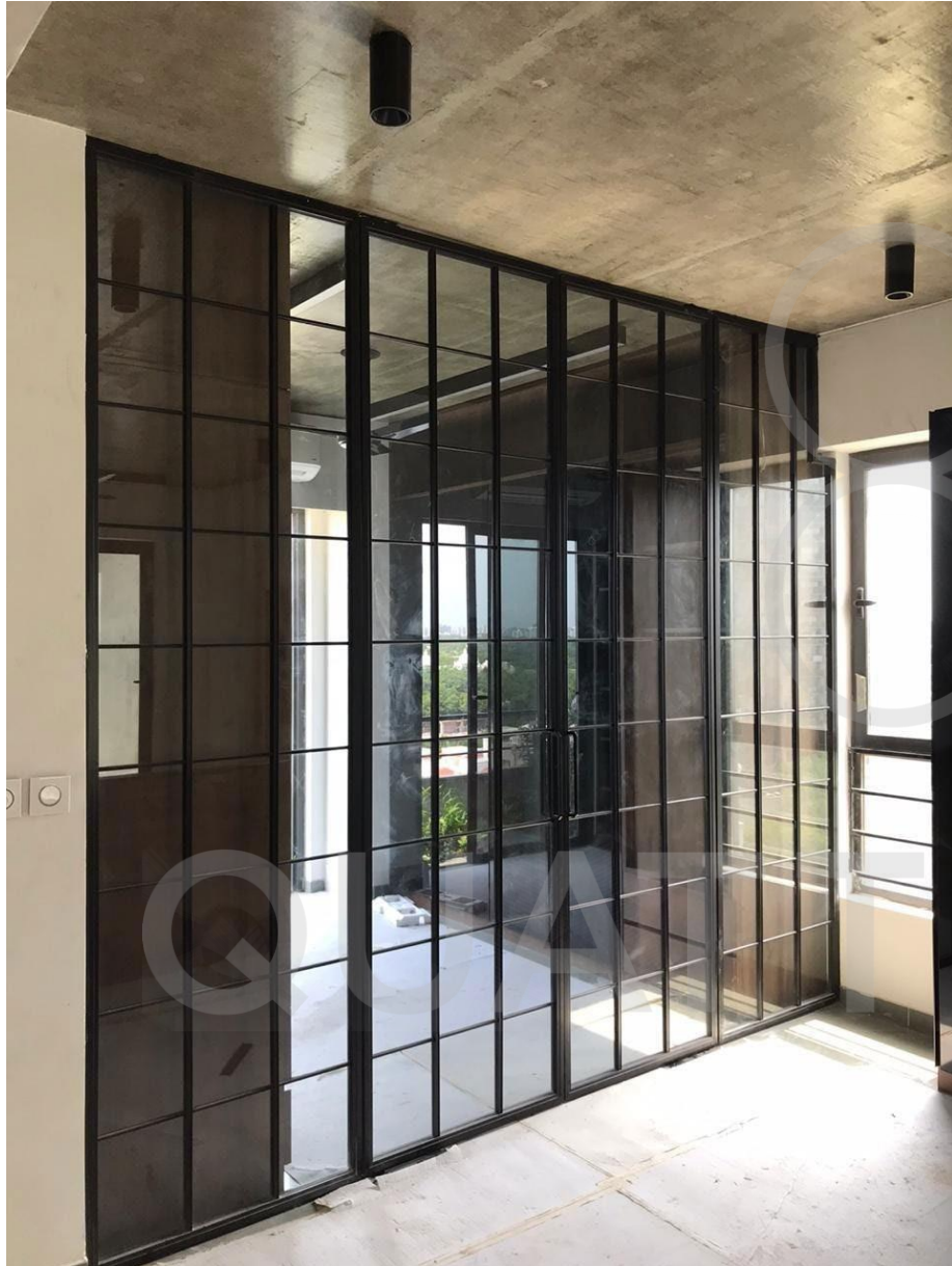
FIXED PARTITION WITH SWING DOOR IN GRIDPATTERN
