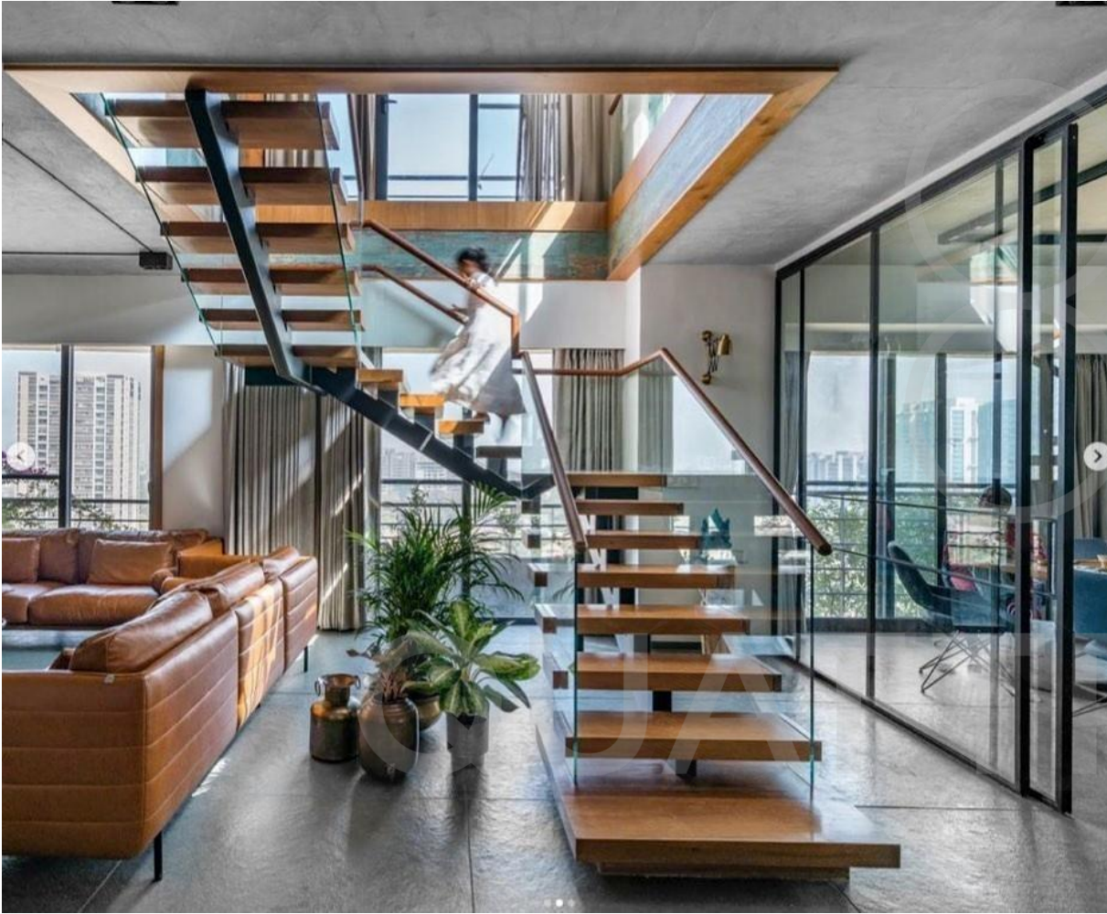
WOODEN STAIRCASE WITH ALUMINIUM AND GLASS RAILING IN WOODEN FINISH
