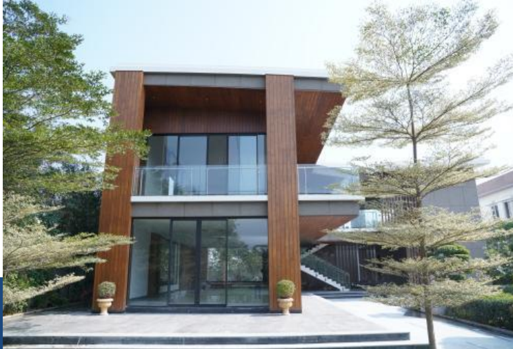
RSV Infra - Urban Village - Clubhouse Hyderabad, India
